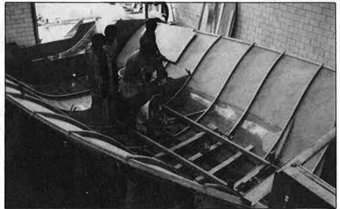
Keel frames and ply bulkheads were fitted and glued.
