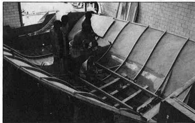
Keel frames and ply bulkheads were fitted and glued.
