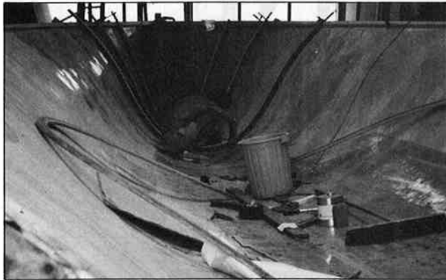
Laminated frames, made earlier, were glued in place.
