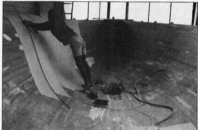
African Ash veneer was laid on exposed interiors.
