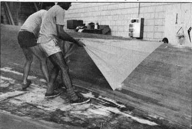
Peel ply was torn off by hand when epoxy cured.
